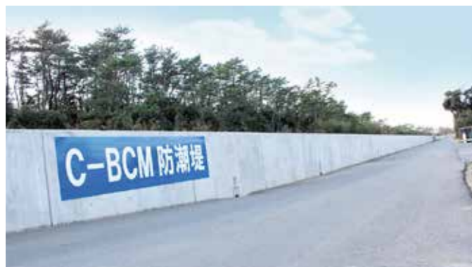
Breakwaters for tsunami countermeasure
